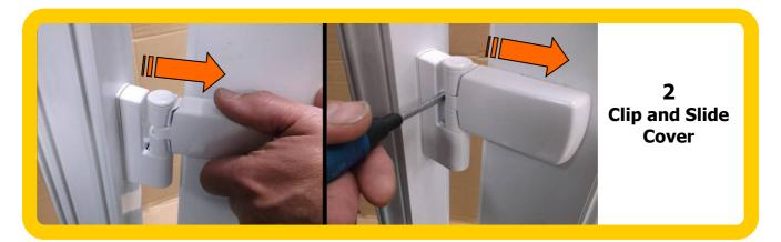
Pull the cover out towards the centre of the door. On release a click will be heard. If the cover does not open by hand a screw driver can be used behind the knuckle to gently assist opening. Repeat stages 1 and 2
